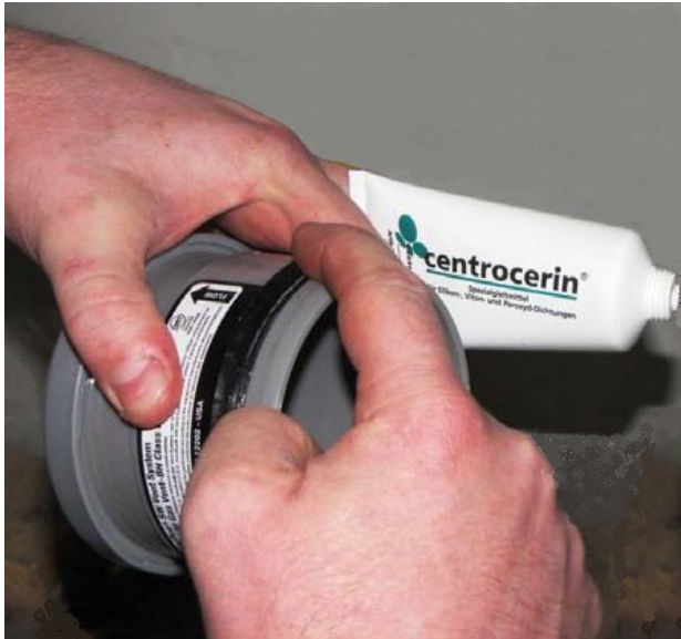
Applying Lubricant to Gasket
